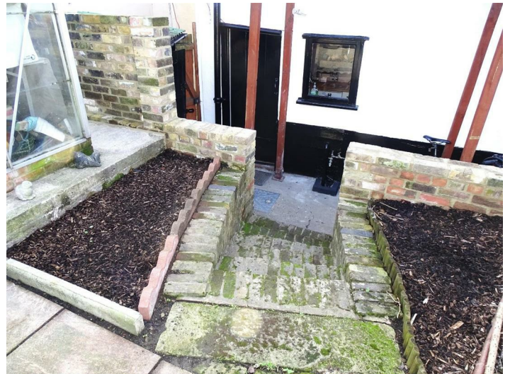
STEPS DOWN TO KITCHEN DOOR
